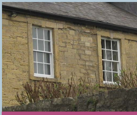
Late 17th Century window heads on the rear elevation of the Manor House.
