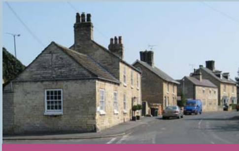
The historic pattern of house, croft and toft survives along The Village and gives a distinctive character to the layout.
